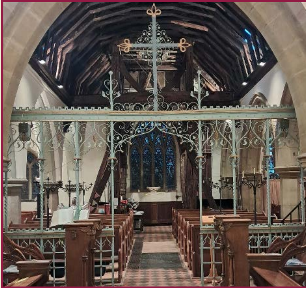
The blue painted iron rood screen above with twisted standards and decorative scroll work is dated 1930.
